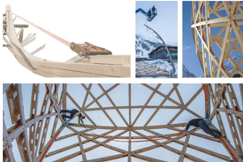
Fig 07: Collage of the bent edge beams of the Neuschneewolke-Lüsens during the production and assembling process. The tension cables are removed in the final configuration; Photos W. Klasz
