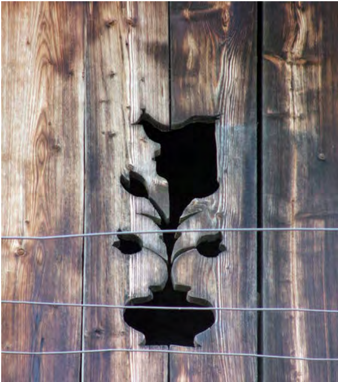
Pic.3 hole for natural ventilation of an attic, foto, Tyrol 2005
