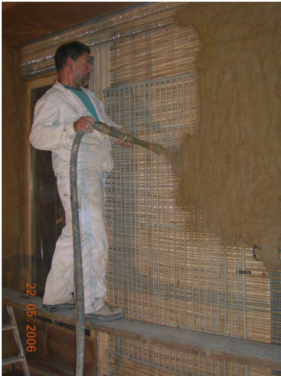
Pic.9 Haus Schönwies, loam rendering above wall heating (solar generated), Tyrol 2006, foto by w. Klasz, design and supervision by w. Klasz
