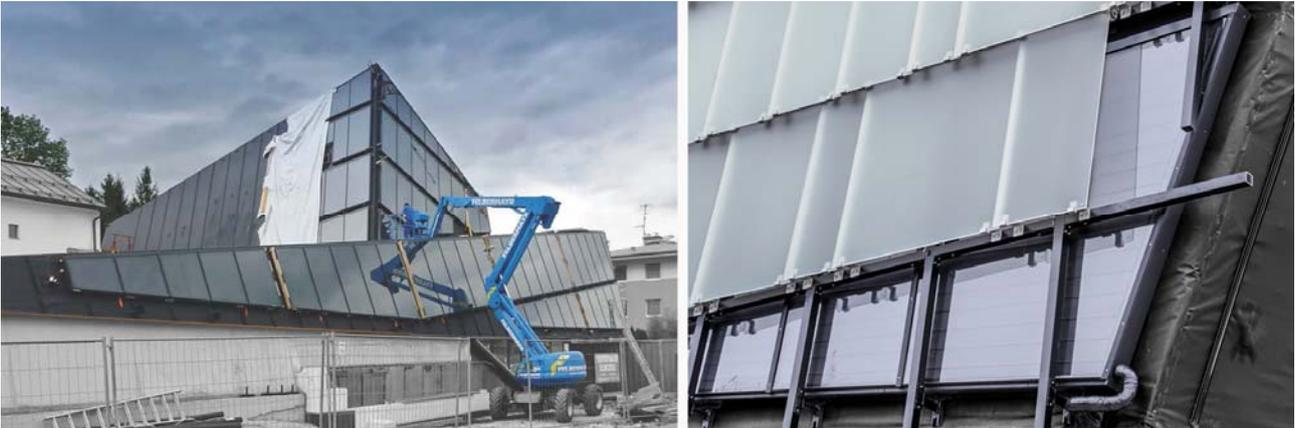
Figure 6: Customized solar panels and the continuous glass layer above the hole building during installation
